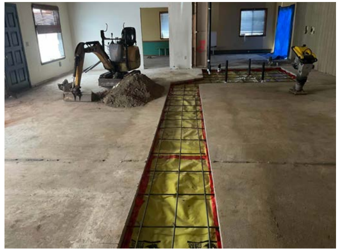
Rebar and vapor installed ready for Concrete
