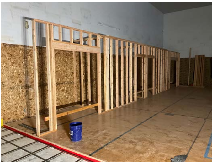
Interior Framing begins for Storage Rooms by the Lounge
