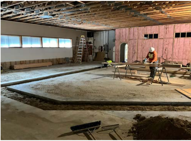
Sewer Trenches Backfill Complete
