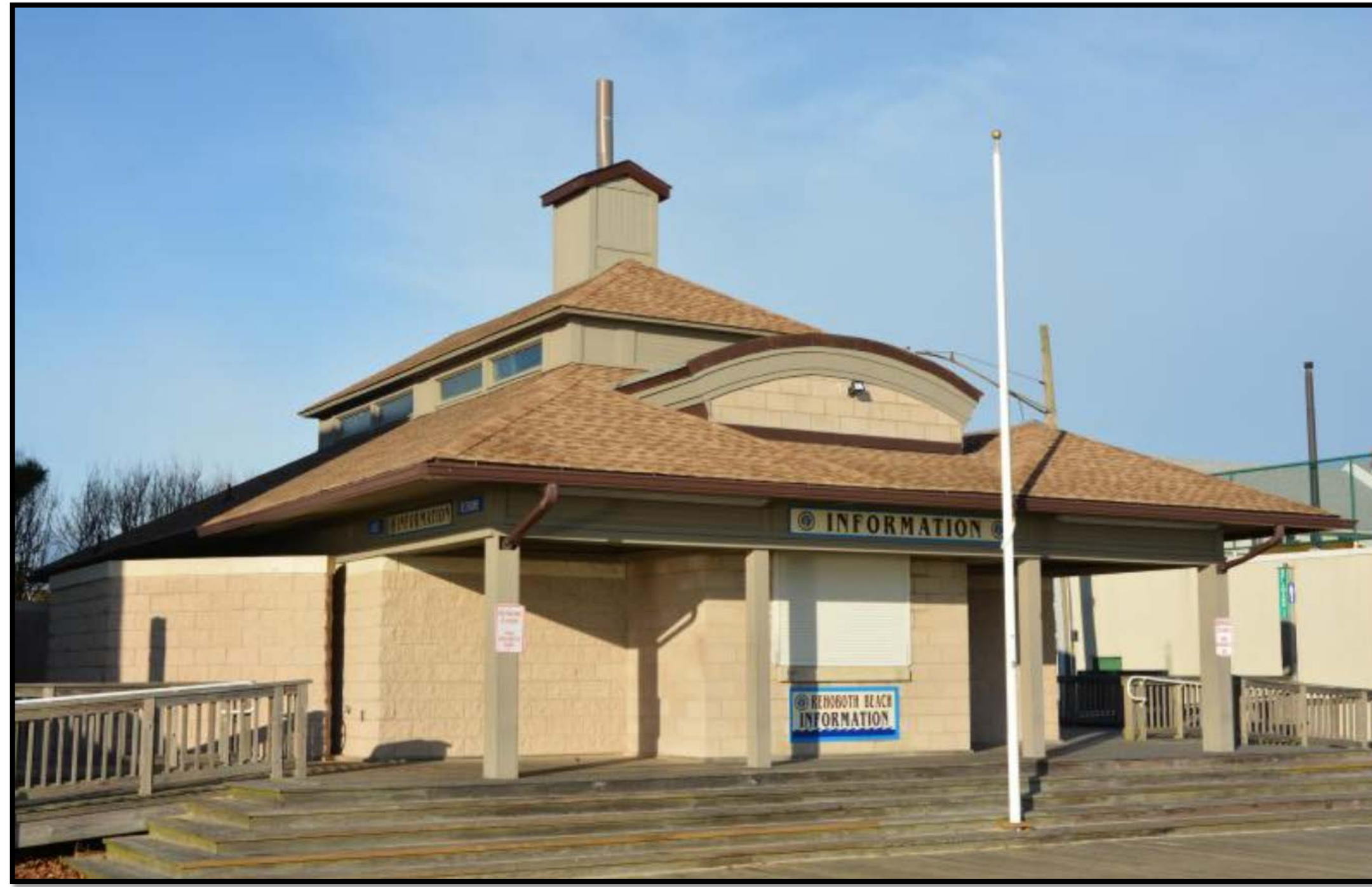
Image Source: https://www.capegazette.com/article/five-att-cellphone-towers-installed-rehoboth/171309
