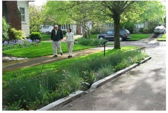
Figure 14.4: Siskiyou project in Portland, Oregon uses traffic calming designs to manage stormwater. Note curb cuts that allow stormwater to enter bioretention area in narrow section of road. Source: Kevin Robert Perry 2005
