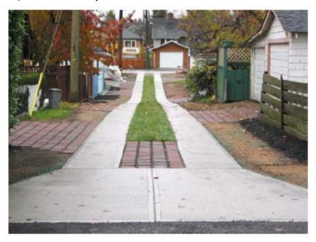
Figure 19.1: Country Lane Alley in Vancouver, B.C. uses a combination of concrete wheel strips, pervious pavers, reinforced plastic grid with grass, and under-drains to attenuate storm flows and create an aesthetic design objective. Photo by Curtis Hinman
