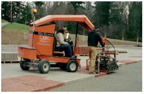
Figure 4.2: Mechanical setting of pervious pavers – Source: Mutual Materials 2008
