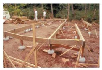
Figure 20.2: A house construction project using minimal excavation foundation pier system.
