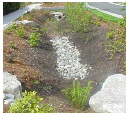
Figure 14.3: Seattle SEAStreets bioretention swale receiving sheet flow from sidewalk and street
