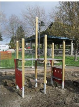
Old playground equipment has been removed. Contractor discovered a thick concrete base under the rubber fall-surface. This was not detailed in the 1991 site plans. Therefore more concrete was removed and additional drain rock and Fibar fill is needed to match the surrounding concrete walkway.
