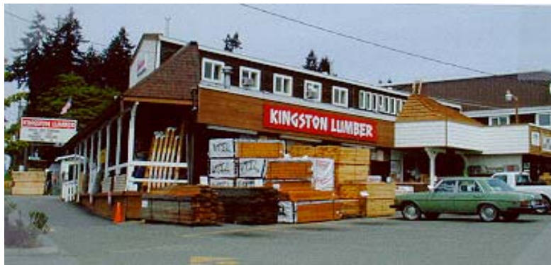
Figure II.A.1.(h). Rural communities need businesses with outdoor sales areas, such as nurseries, lumber yards, hardware stores, and feed stores. Outdoor sales and storage areas can harm a business's and community's identity if not handled in an attractive manner. The two positive examples in this figure solve this problem in different ways. Sack's Feed and Garden Store provides an attractive landscape screen and display, while Kingston Lumber incorporates a covered sales area. In both cases, the parking is located at the side of the building. Note how both businesses are inviting assets to the community's character. Also note how Sack's sign is modest but attractive and ideally located for maximum visibility.
