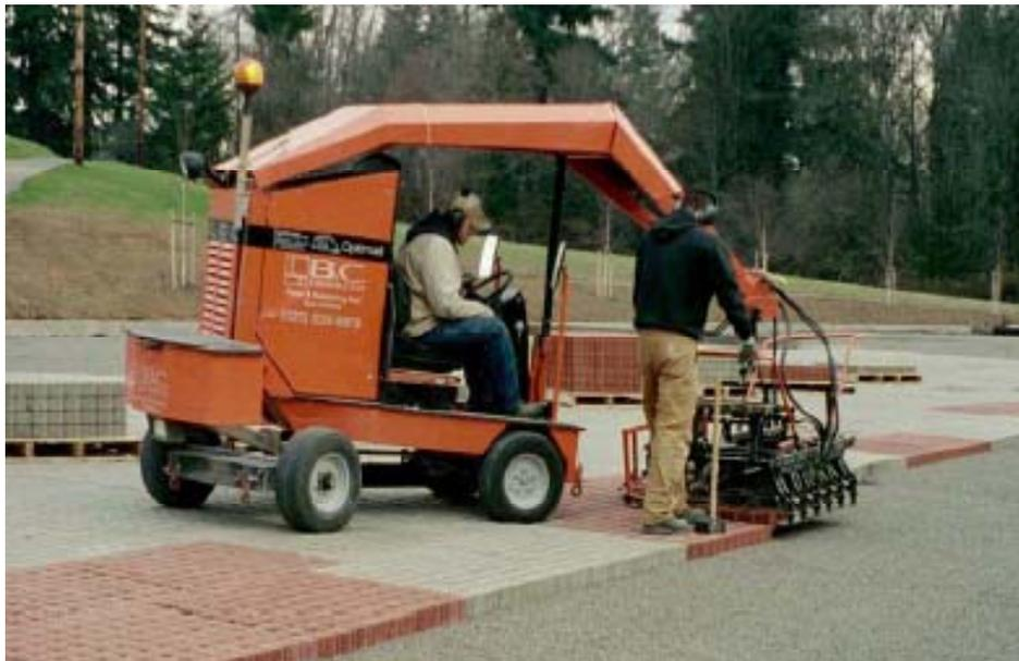
Figure 4.2: Mechanical setting of pervious pavers – Source: Mutual Materials 2008
