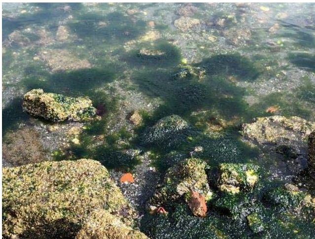
Photograph 3. Sea lettuce at the base of the riprap revetment.
