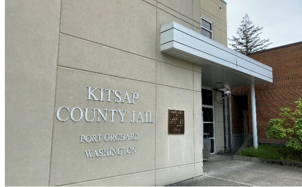
Kitsap County Jail Entrance
