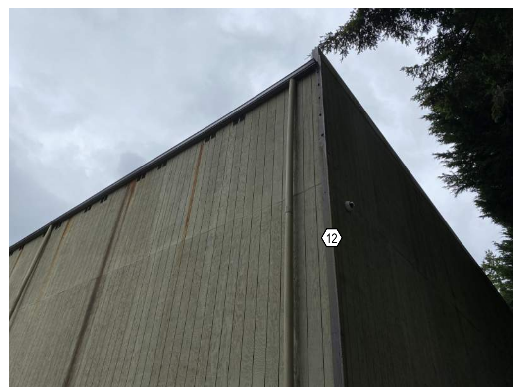
3 NORTH FACE AT UPPER WEST CORNER 1" = 1'-0"
