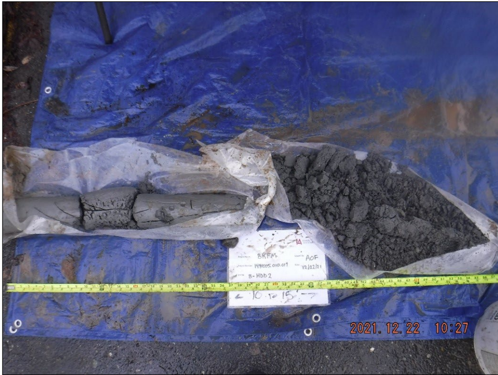
20. Boring B-HDD2, 10 to 15 feet deep.
